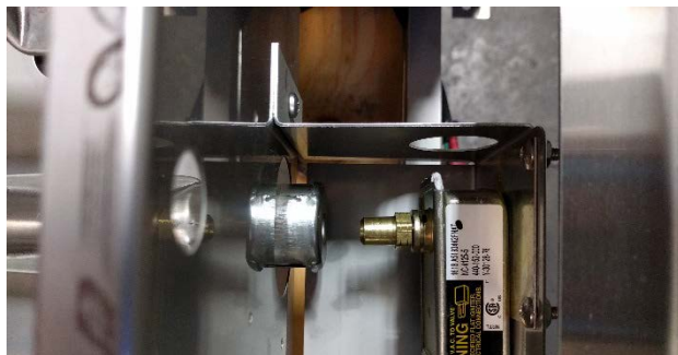
INCORRECT INSTALLATION THE ORIFICE IS OUT OF POSITION AND IS NOT INSERTED INTO THE VENTURI
