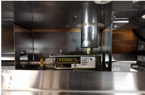
CORRECT INSTALLATION THE ORIFICE IS COMPLETELY INSERTED INSIDE THE VENTURI
